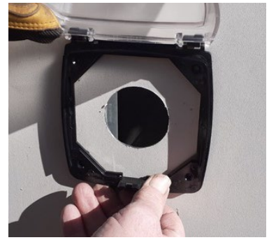
Measure cover and mark where screws are to be installed. Install foam water proofing gasket between mount and HVAC unit. Use self-taping screws. DO NOT OVER TIGHTEN
