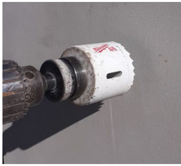
Drill 2-inch hole in duct or HVAC unit.
