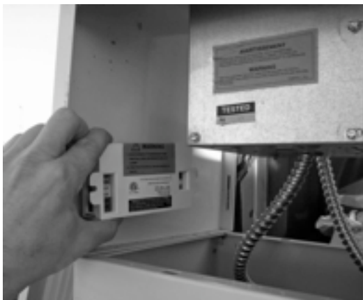
Example of HVAC electrical box mounting
