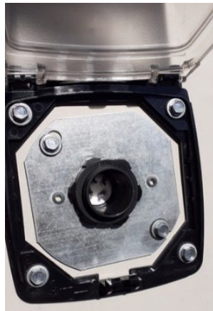
Install mount assembly with 2 self-taping screws.
