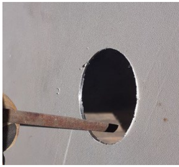
File sharp edges to avoid injury or damage to the lamp wires.
